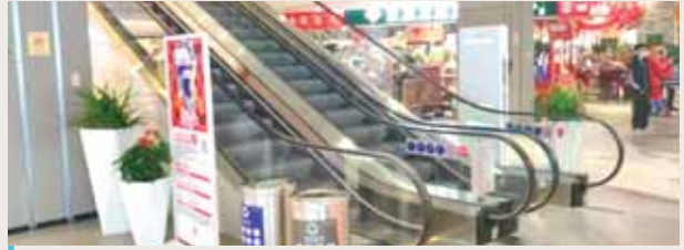
Installation of additional set of escalators
