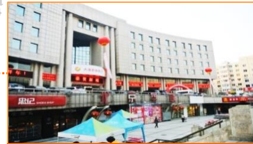
Dalian Jinsanjiao Property
